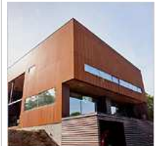
In Japan, a House of Steel
