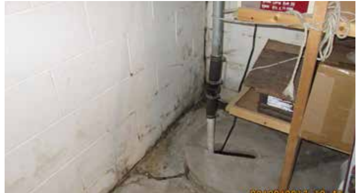
Figure 1: Basement Leak
