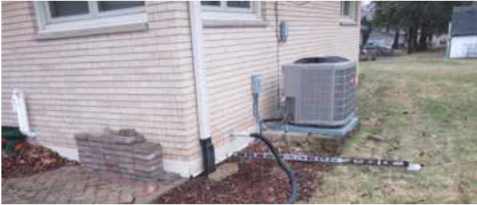
Figure 4: Exterior Grading, Downspout, Pump Discharge
